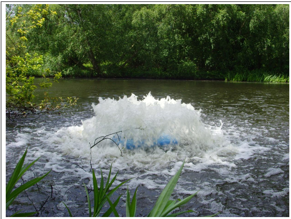
Splash Mixer in operation
